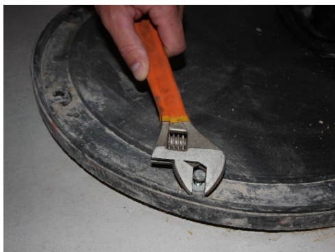
STEP 1 Remove sump pit lid.
