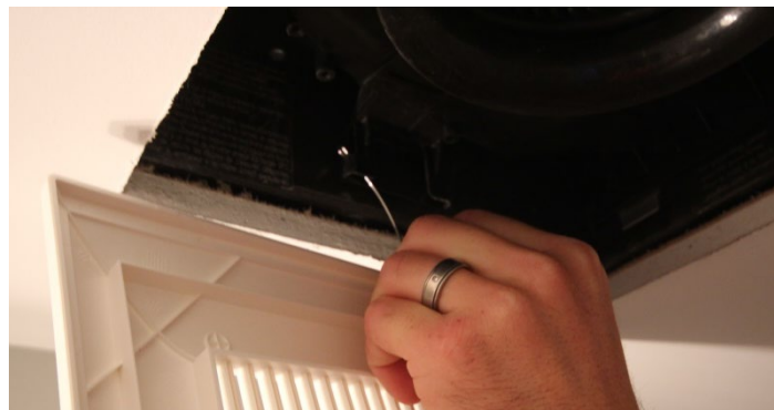
STEP 3 Remove cover and inspect / clean fan turbine.
