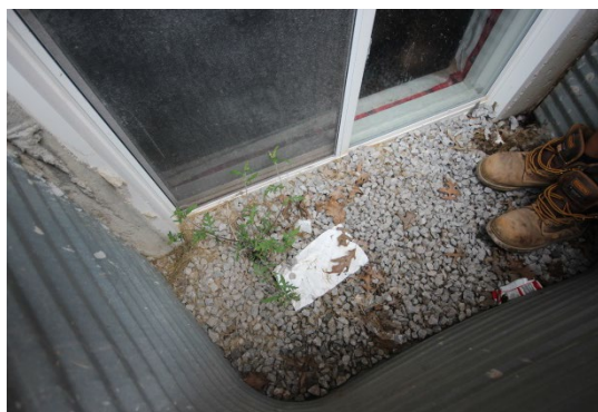
STEP 1 Remove leaves, dirt, garbage, etc.
